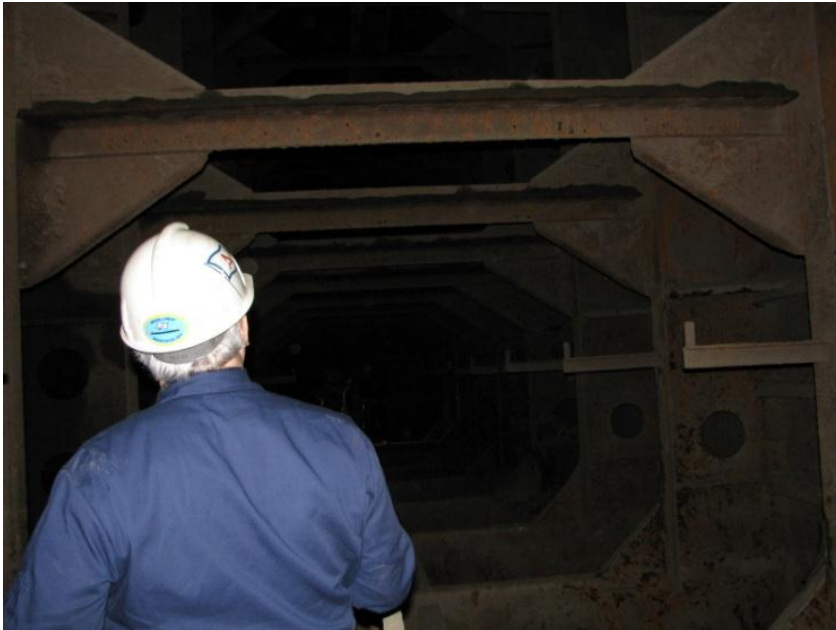
Inside a ballast tank on the M/V Indiana Harbor
